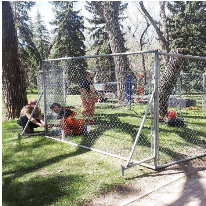
City of Moose Jaw crew assembling fence around one of the trees to be carved.
